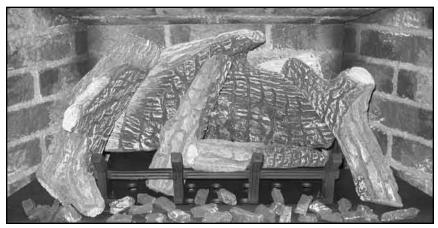
Figure 28. Fourth Stage Log Set Installation.
